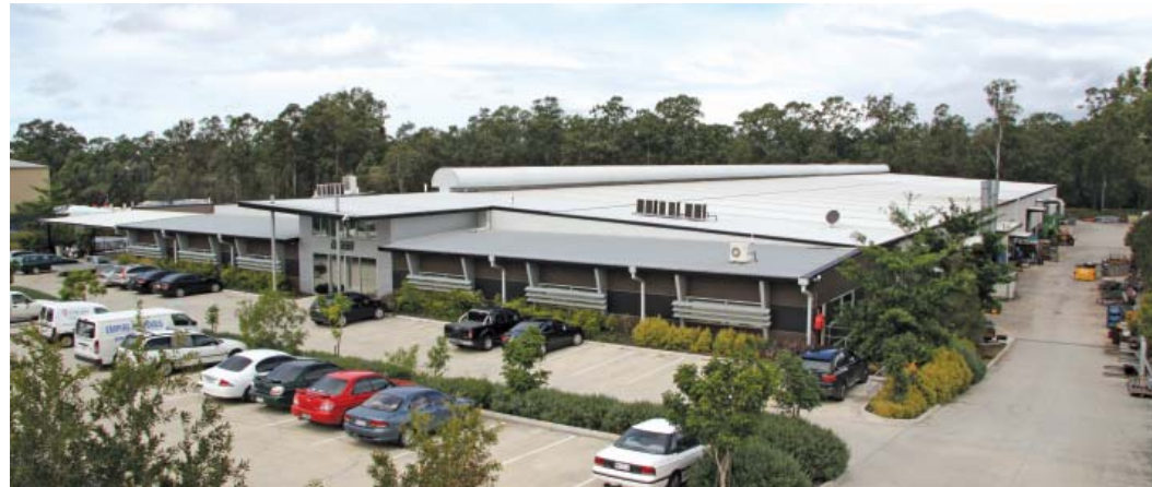
Digga's 12,500m 2 (130,000 sq ft) state of the art manufacturing facility, Brisbane Australia.
